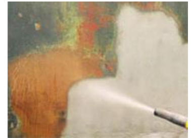
SAT Blast in operation cleaning metal and brick
